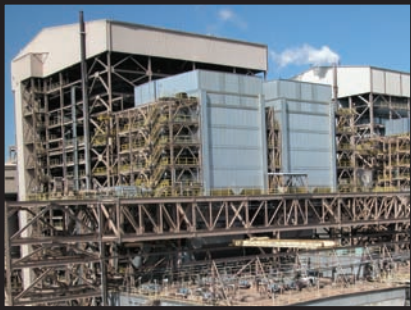
Installation of SCRs photo courtesy of Babcock Power
