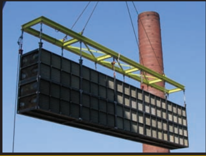
Plate Type Catalyst for Horizontal Flow SCR photo courtesy of Argillon
